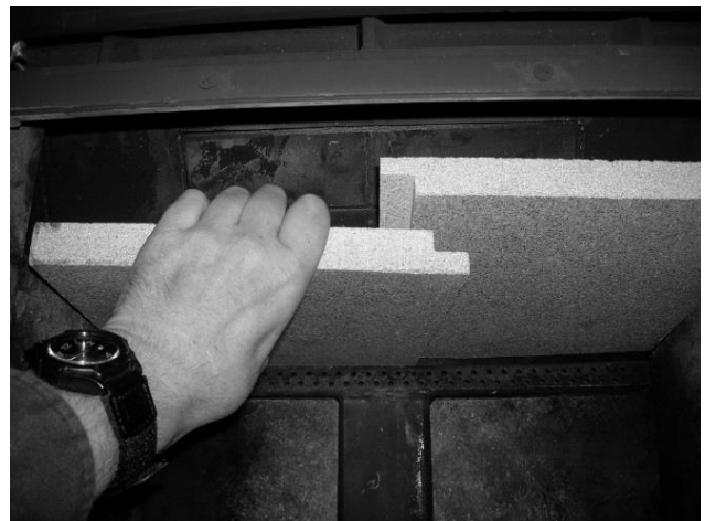
Figure 16 - Removing/Replacing the Baffle for Inspection
