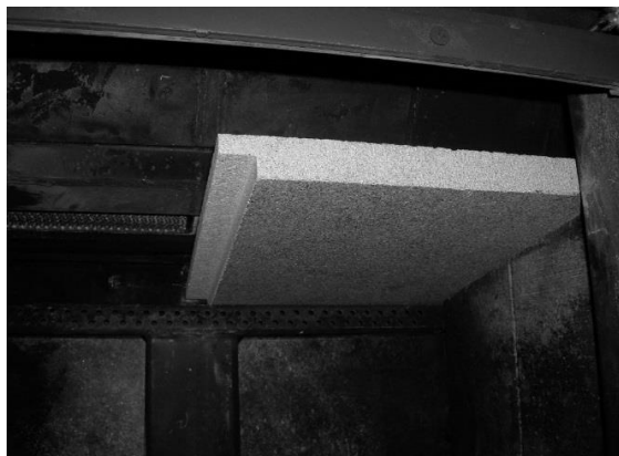
Figure 186 (cont.) - Removing/Replacing the Baffle for Inspection
