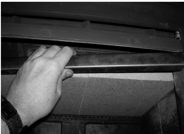
Figure 16 - Removing/Replacing the Baffle for Inspection
