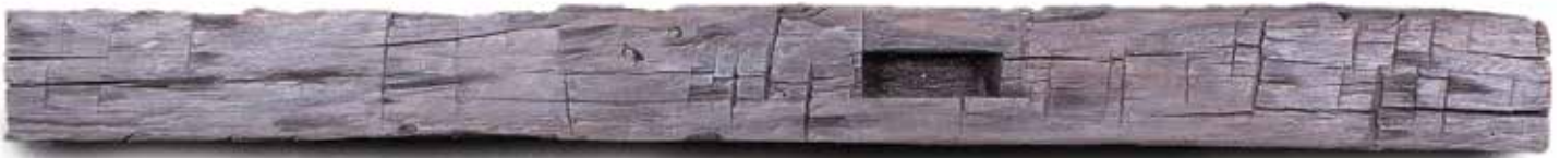
Hewn Mortise Beam
